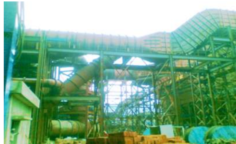
Process Gas Ducting • JSPL Barbil-Pallet Plant
